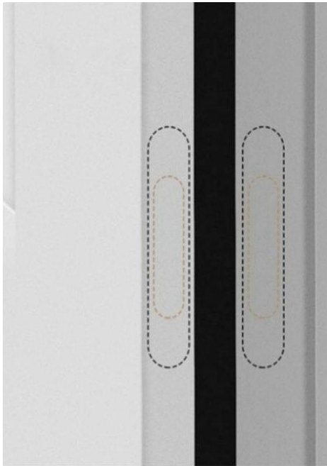
① Draw the installation position
